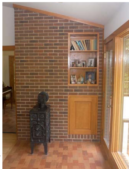
Thermal mass, like this brick wall and floor, stores solar heat and releases it slowly.
