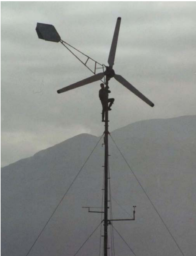
This LMW has a diameter of 5 meters. With its large rotor and tall tower, it is ready to catch the slightest wind.
